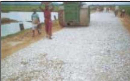
Dry compaction of metal and application of screening material: Narbari Road, Assam.
