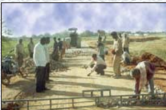
Laying of metal with the help of Camber Board: Length: 4.20 Km. Cost 64.56 Lakhs. District Gwalior, Madhya Pradesh.
