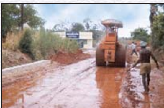
Laying of metal with the help of Camber Board: Length: 4.20 Km. Cost 64.56 Lakhs. District Gwalior, Madhya Pradesh.
